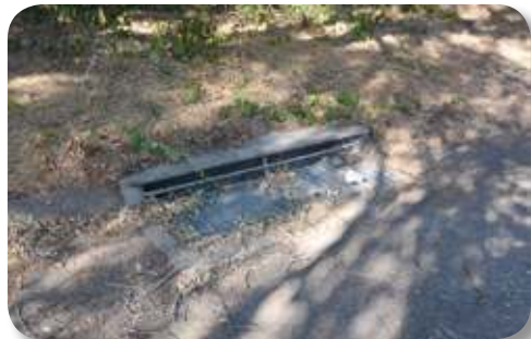
Leaves and debris can clog drains and cause flooding. Clear drain areas around your home before the rain starts. Check curbside gutters and drains and, if they are clogged, alert local officials or other responsible parties.
